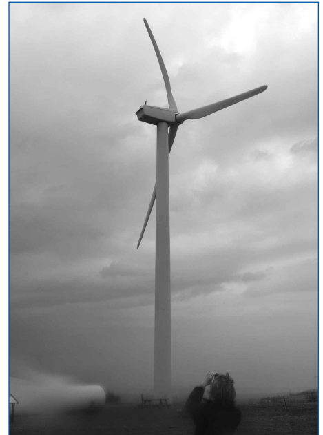
Close-up of a wind turbine on the Fenner Wind farm, as seen during a recent tour taken by New York AREA
